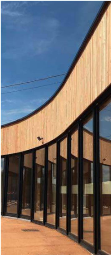
Ensemble chassis bois/aluminium Gugnécourt
